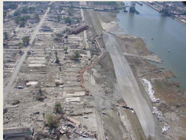
Sheet pile walls and floodwall collapse
